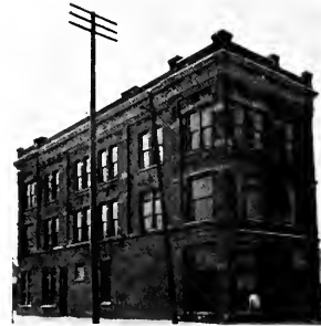
FIG. 18.—REPEATER AND SWITCHING STATION, TOLEDO, OHIO.
